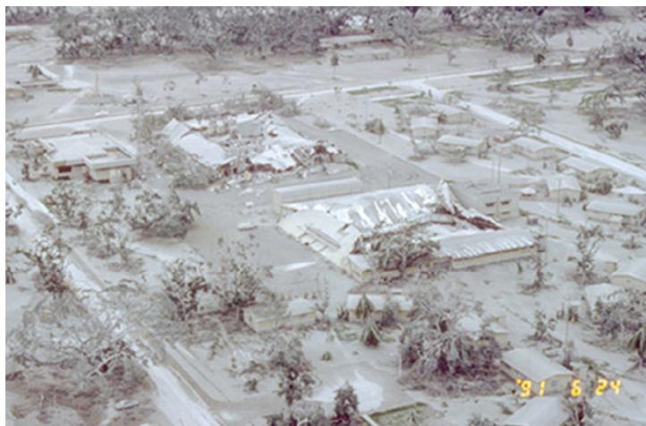
Figure 5. Ash-fall damage to rooms at Clark Air Base, ~25 km east of Pinatubo (Philippines). The photograph is in true color (courtesy of W.E. Scott, U.S. Geological Survey).
